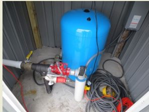
Irrigation Well Pump and House
